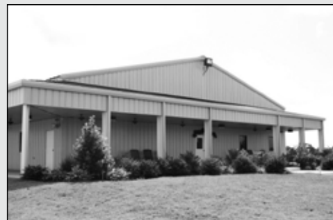
Wiggins Sale Facility
