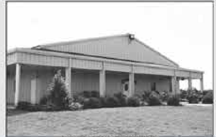
Wiggins Sale Facility
